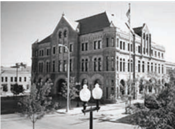
US District Courthouse, Sioux Falls, SD
